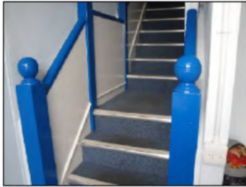
Figure 57 – The inserted stairs from second floor level up into the c1920s roof extension.
